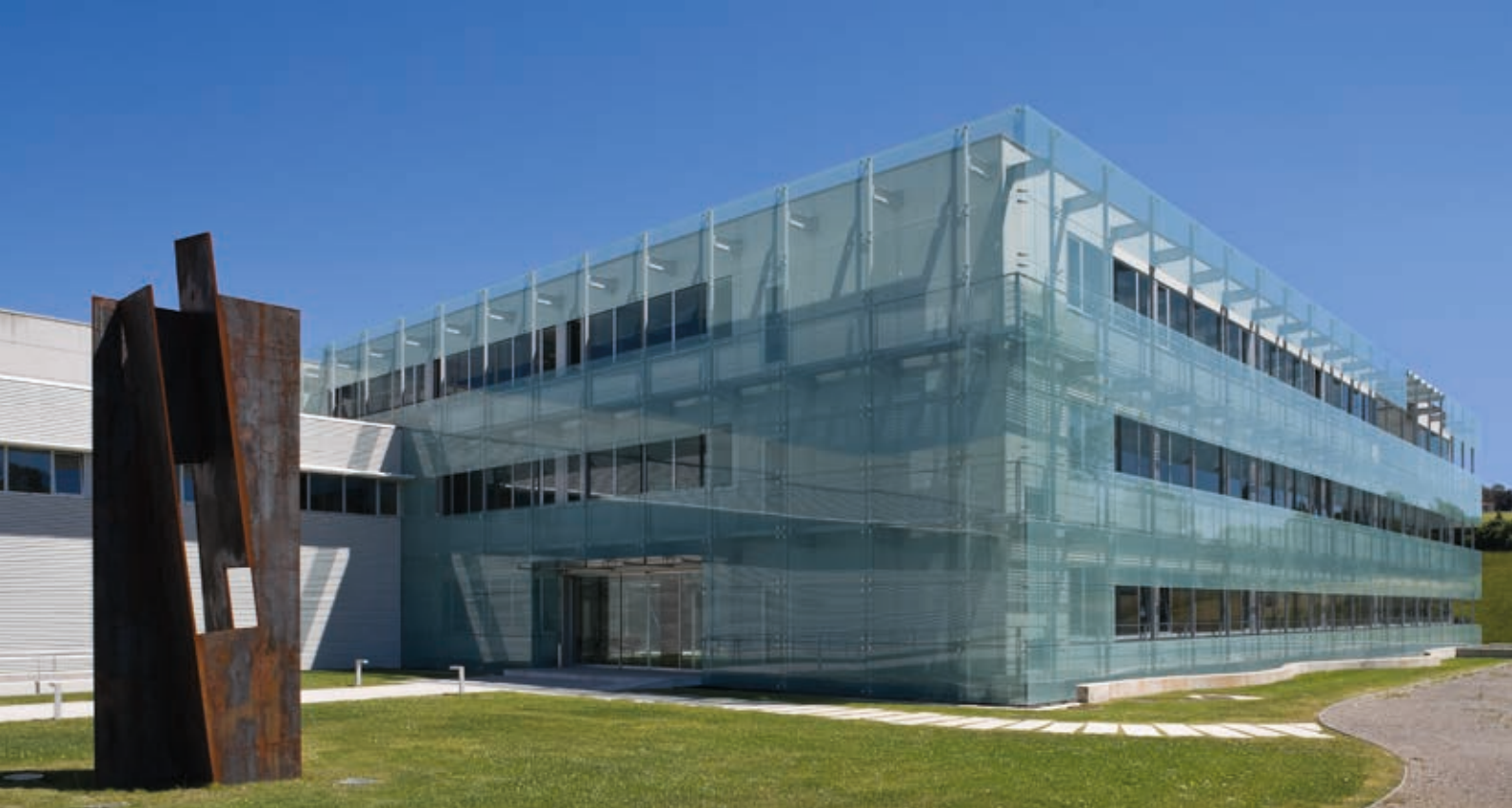
Headquarters Offices and Technical Centre in Gijón (Spain)
